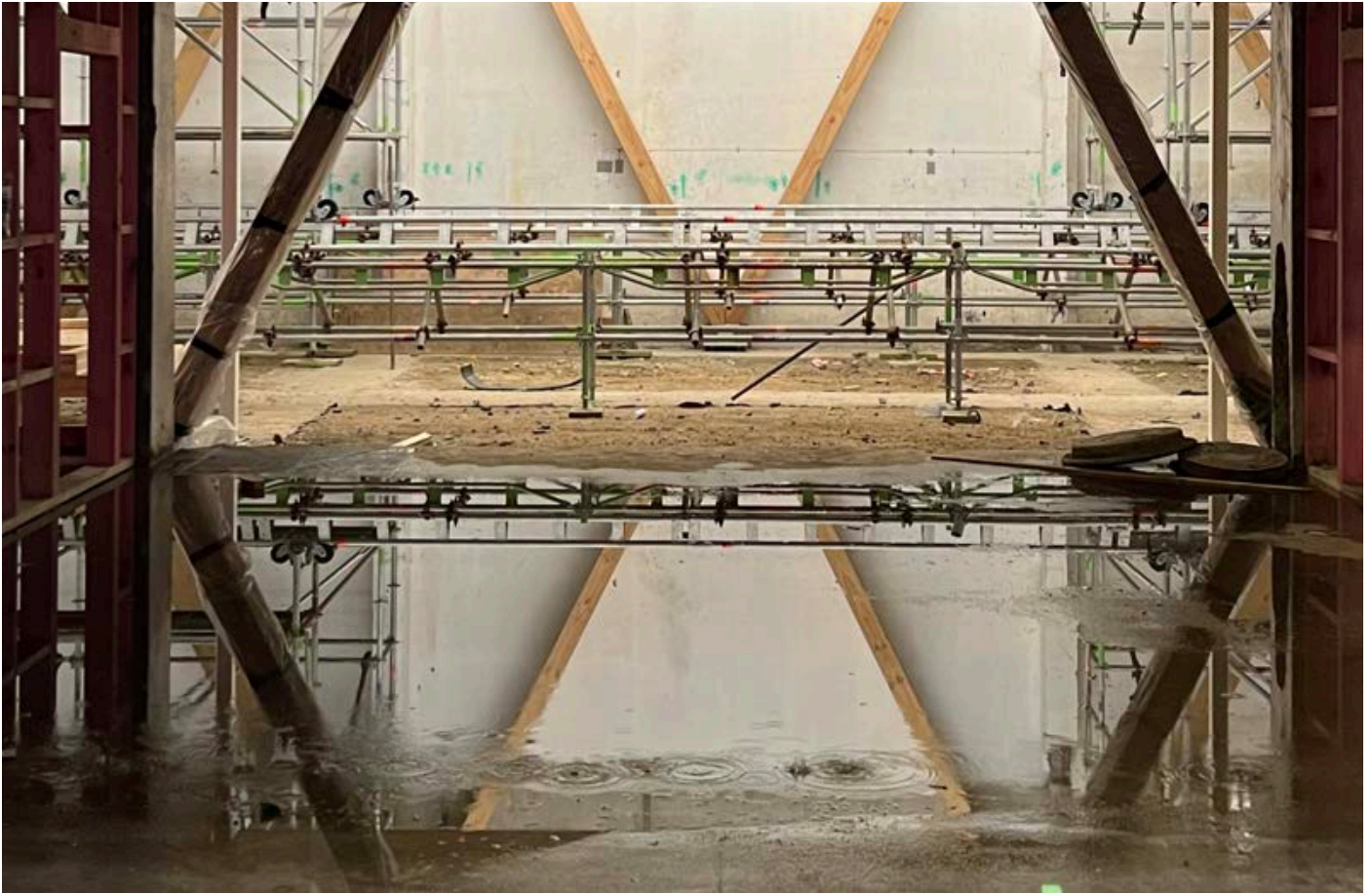
Arcade from below under construction (looking east)
