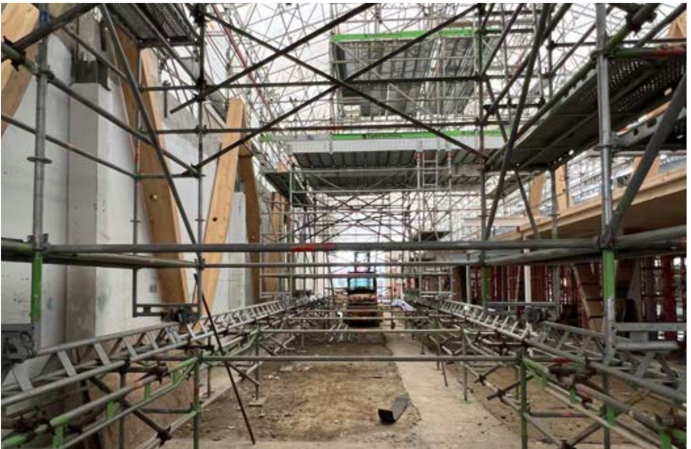
Arcade under construction (looking south)
